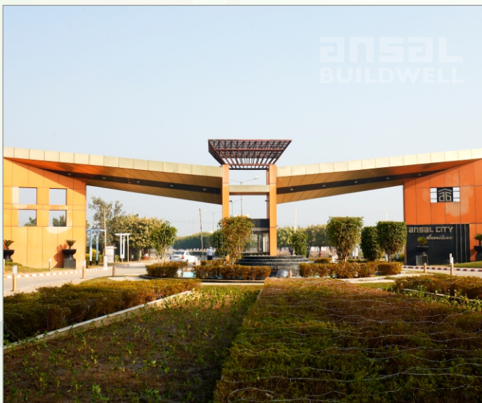
Actual site photo of Entrance Gate
