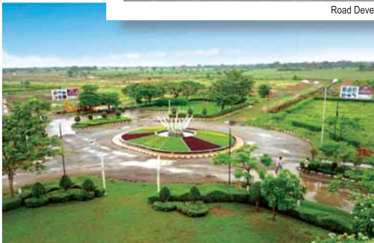
Aerial View of Block E Ansal Basera City Jhansi
