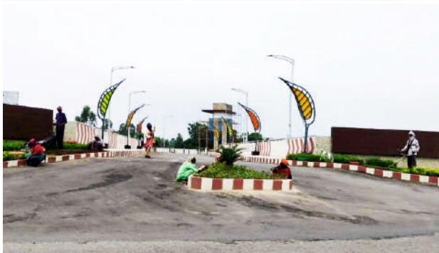
Bridge & Entrance Gate at Florence City, Pathankot.
