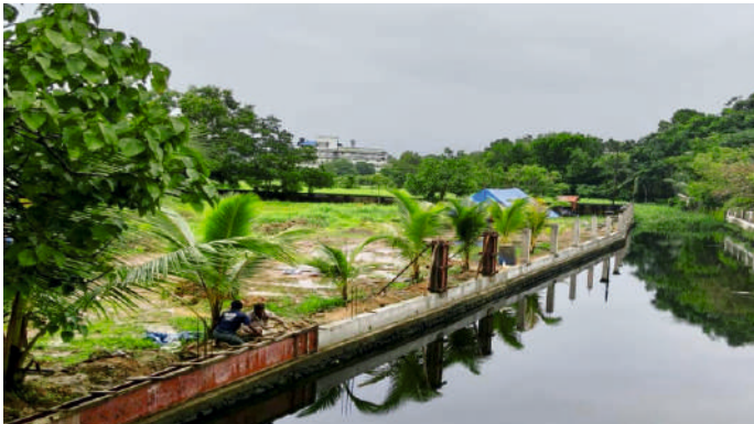
Development work started in Florence Grove, Kochi on the land beyond Thodu
