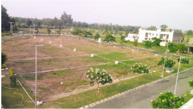
Aerial view of development work at Florence City, Pathankot.
