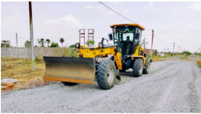
Road work at Ansal Basera City, Jhansi
