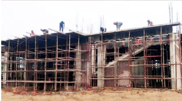
Community Centre under construction at Ansal City, Amritsar.
